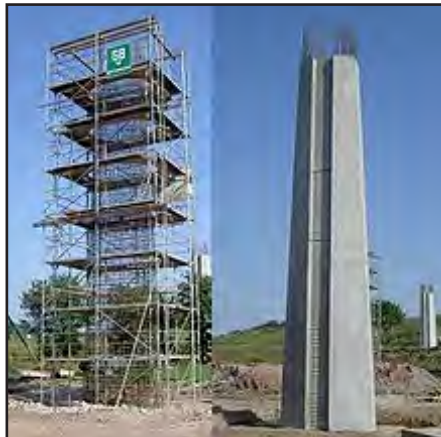
Here is a reinforced concrete column, seen before and after the concrete has been cast in place around the rebar cage.
